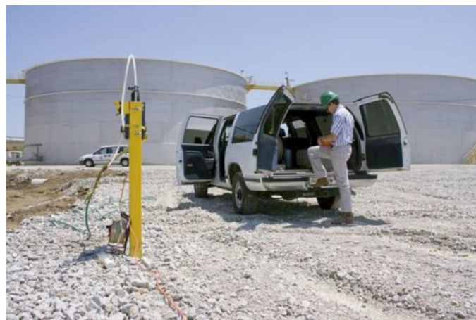
Figure 3-4: Example of a Groundwater Monitoring Well
