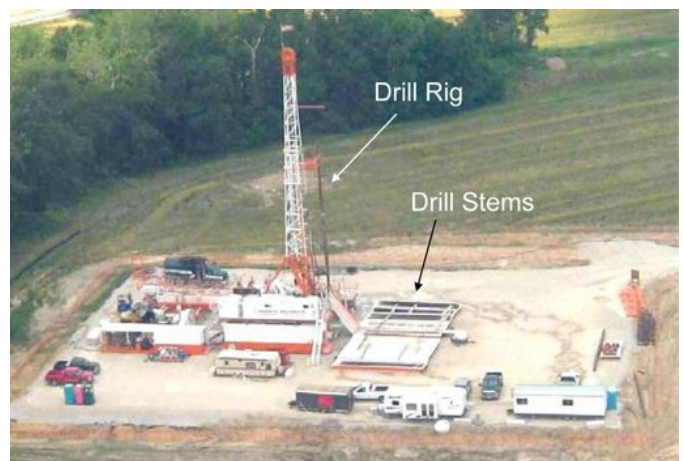
Figure 3-2: Example of a Facility Layout During Drilling
