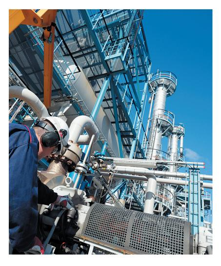
Right: this 30 MW lignitefired steam generation plant was established as a pilot project for the evaluation of carbon dioxide capture using oxyfuel combustion technology. The resulting carbon dioxide is compressed before being stored in geologic formations instead of being emitted to the atmosphere.
