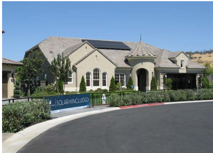
New solar home community in El Dorado Hills. Photo by California Energy Commission
