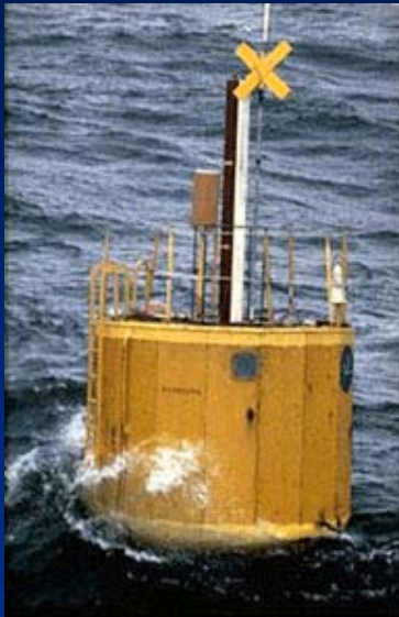
Early prototype, 3 m diameter steel buoy, with glass-reinforced-plastic tail tube, 1 m diameter, 20 m long
