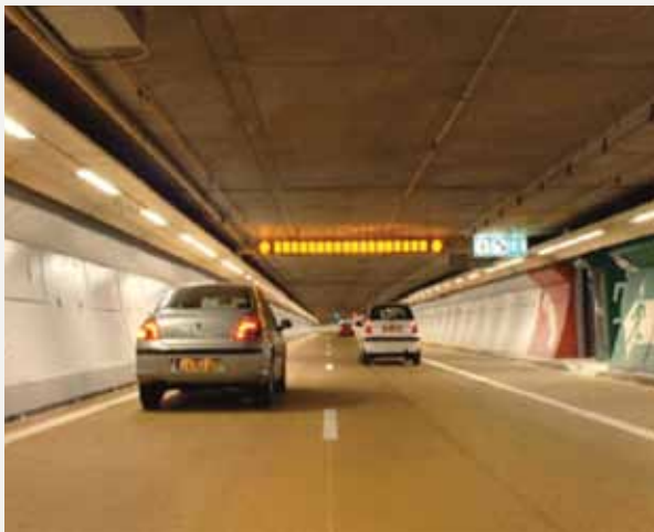
The first toll tunnel has two low-clearance decks and is exclusively for light-duty vehicles. The second tunnel is of traditional style.
