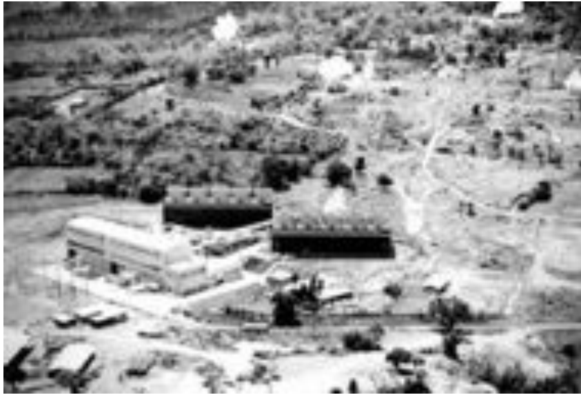
Figure 8.2 Ahuachapan geothermal facility after commissioning around 1977 (DiPippo, 1978).
