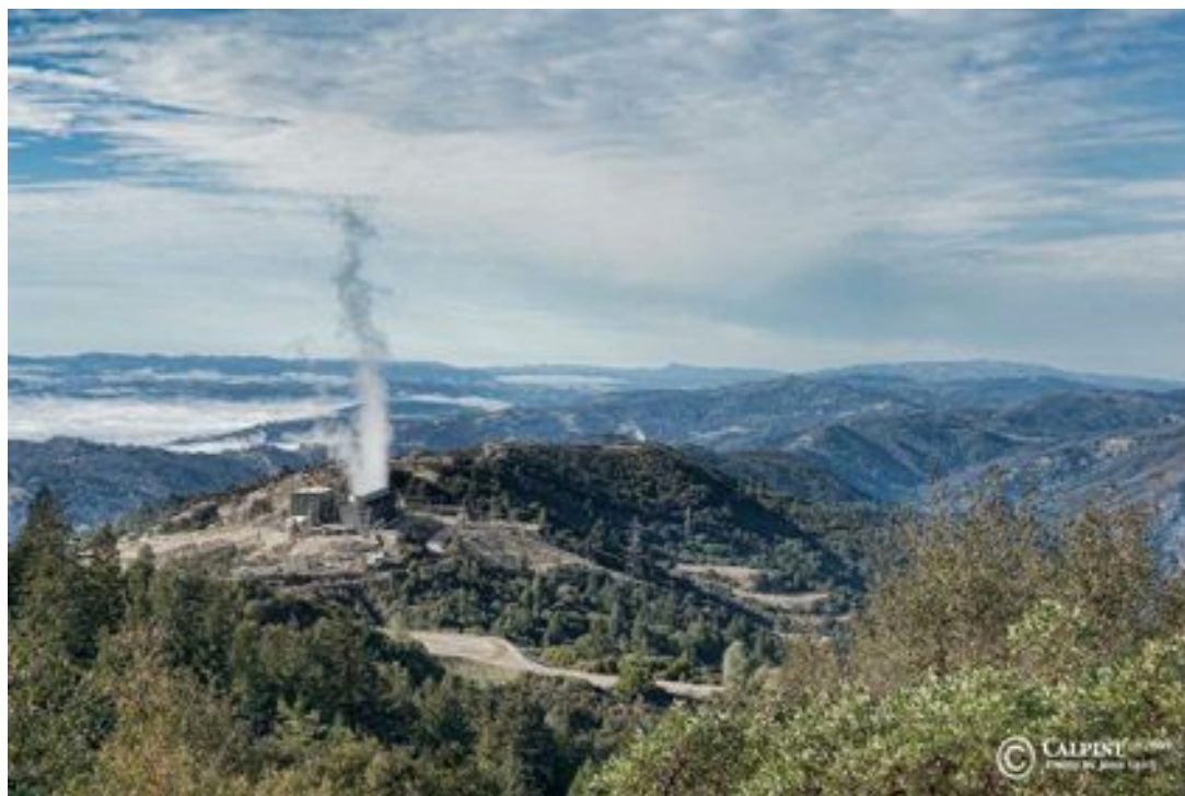
Figure 3.3 Ridgeline Unit 7 and 8 Power Plant (rated at 69 MW) in the left foreground at The Geysers in California. The turbine building, housing the two turbine-generator sets, the operator’s control room and various plant auxiliaries are on the left. The evaporative cooling tower with steam emanating from the top is on the right of the main complex. The beige pipelines along the roads (with square expansion loops) are the steam pipelines that gather the steam from the production pads and bring it to the plant. A high-voltage transmission line (denoted by lattice towers) is in the middle foreground of the picture. SOURCE: Calpine.
