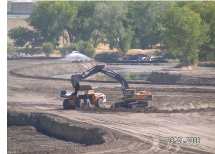
Equipment-intensive construction on 102 Ranch project (Chris Segal, TNC, 2008).
