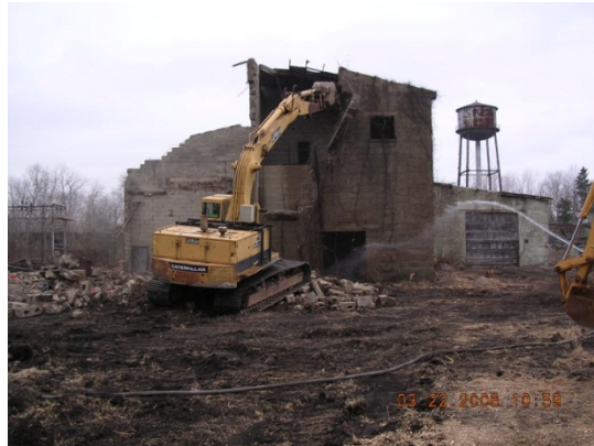
Demolition of mill building and fugitive dust abatement (NPS).
