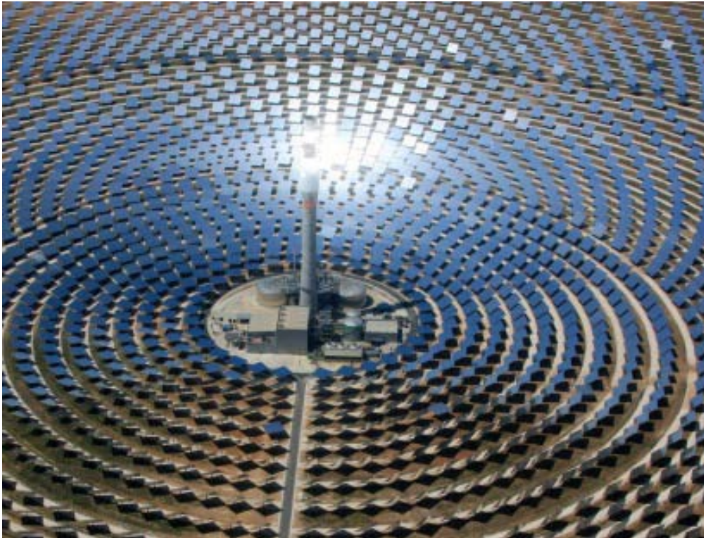
Figure 23: Gemasolar CSP in Seville, Spain with molten salt storages
