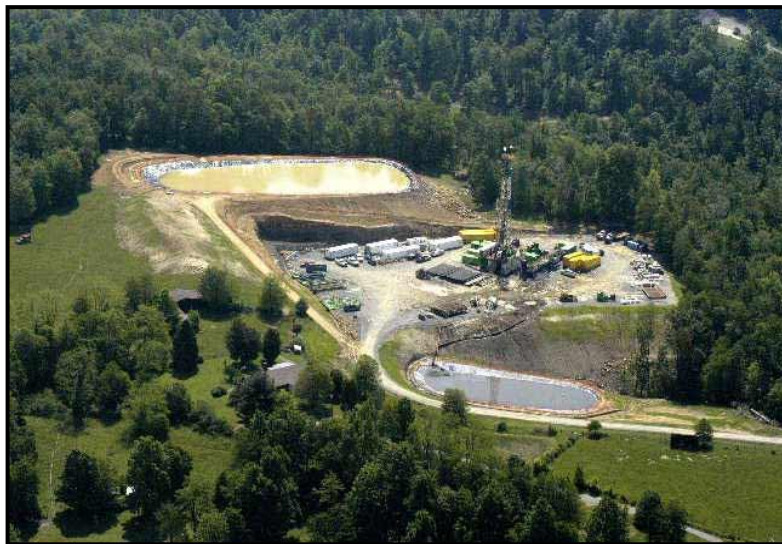
Source: WVSORO Drilling Rig in Rural Upshur County, West Virginia
