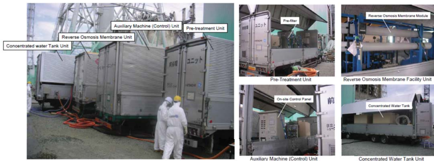
Figure 12. Photographs of portable water cleanup and decontamination treatment units. (Courtesy of TEPCO.)
