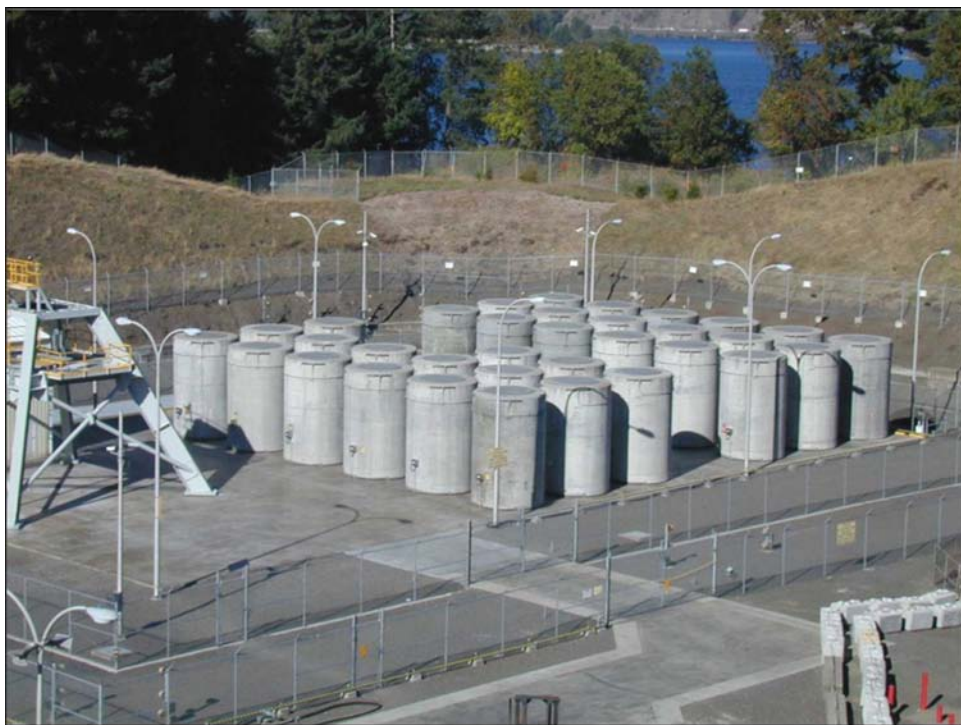
Figure 6: Spent Fuel in Dry Storage
