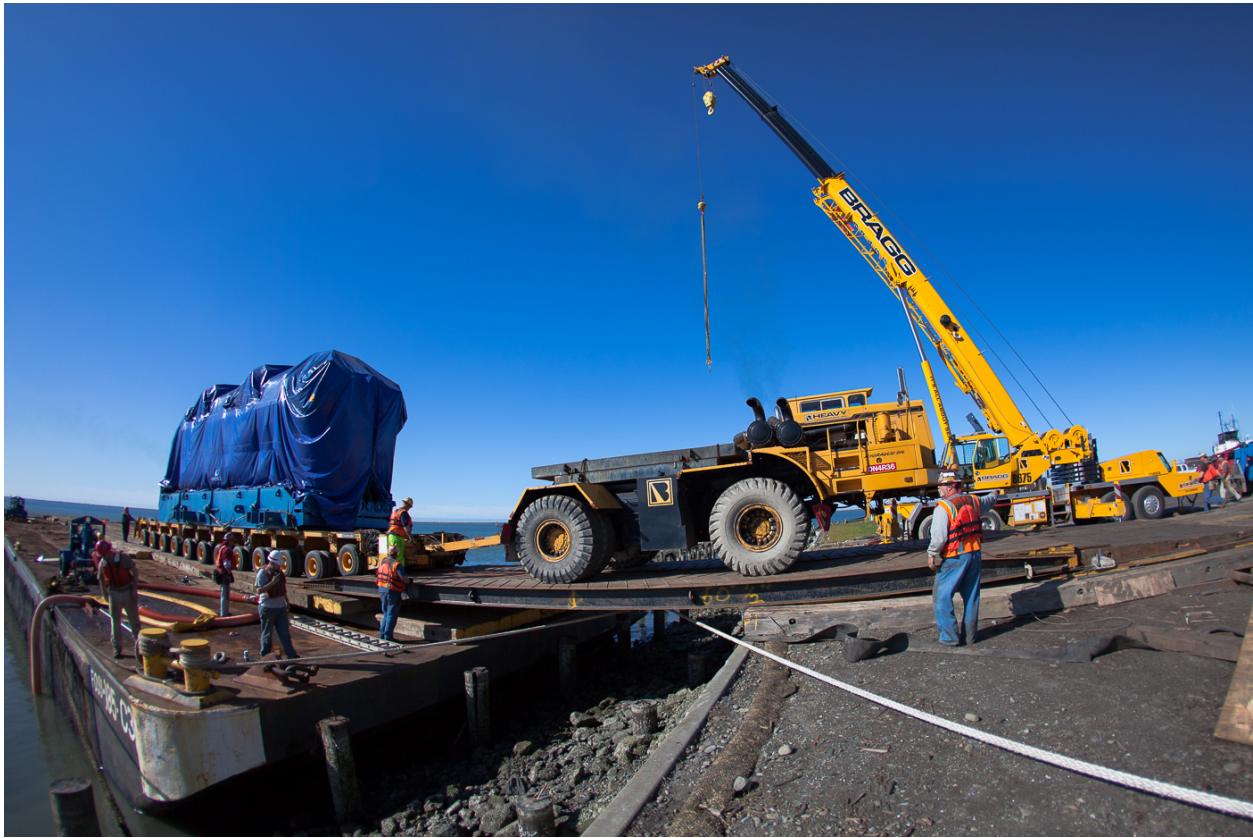
Photo courtesy of Bragg Crane & Rigging Co.
