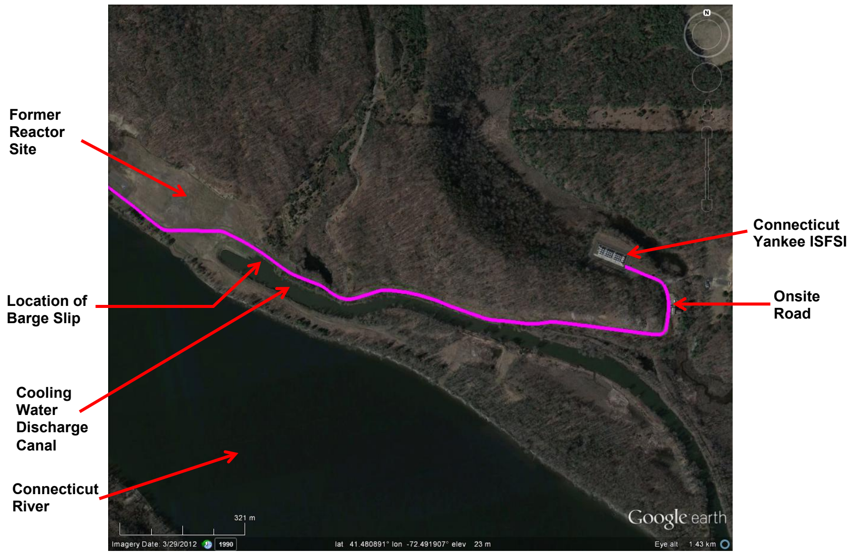
Figure 3-6. Aerial View of the Connecticut Yankee Site (Google 2012)
