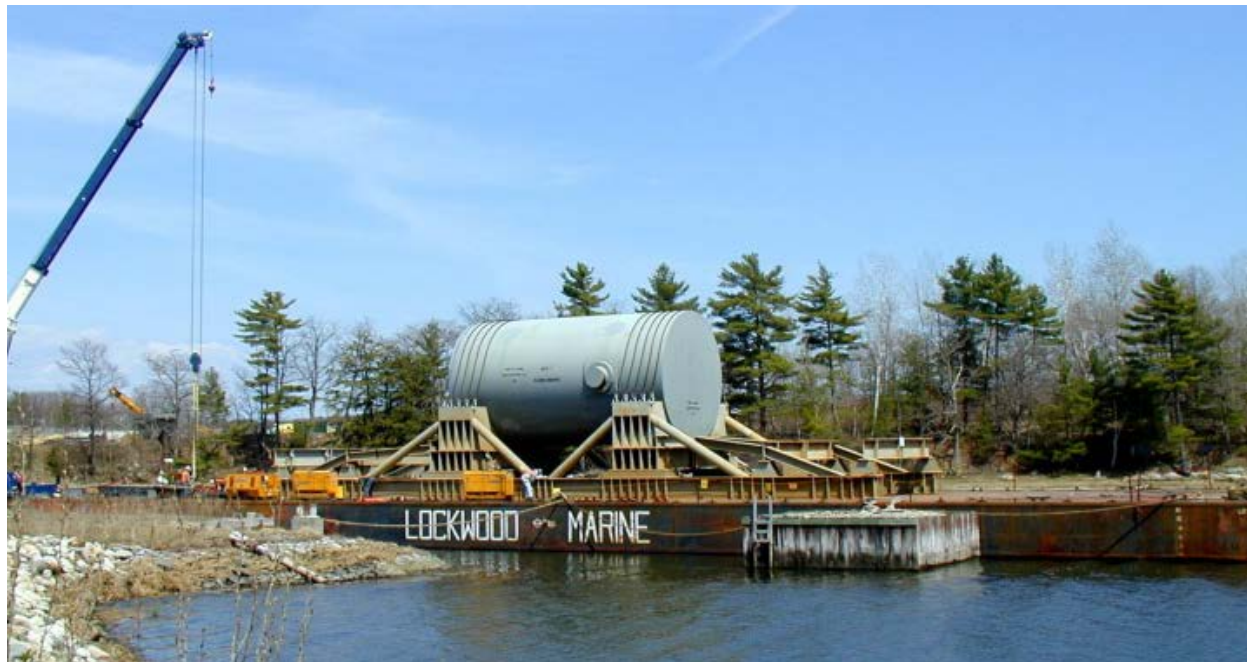
Figure 4-24. Maine Yankee Reactor Pressure Vessel Being Loaded onto Barge
