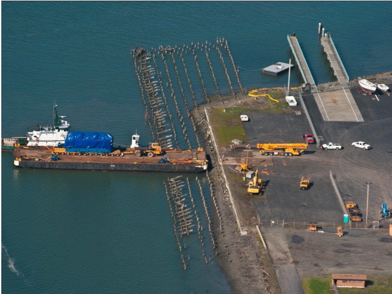
Photo courtesy of Bragg Crane & Rigging Co.
