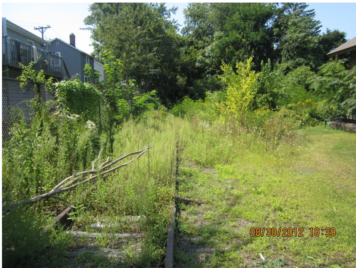
Figure 4-22. Current Condition of Portland Railhead
