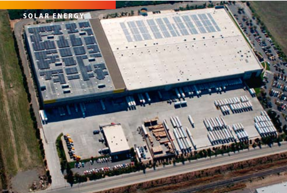
Fig. 5: Distributed solar: Sun-Edison 1 MW PV installation in progress on a Walgreens in Woodland, CA, USA
