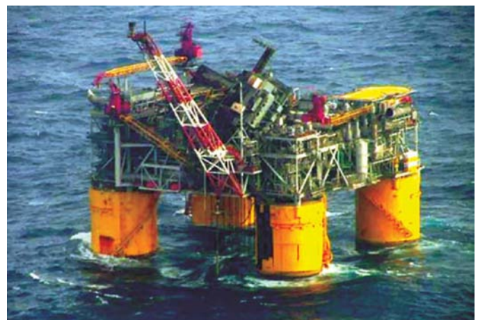
Figure 20. Damaged offshore platform after Hurricane Katrina
