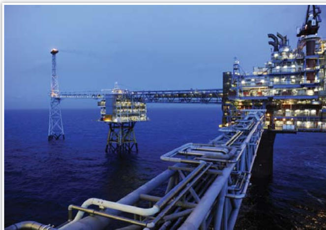
Sleipner in Norway is one of four large-scale commercial CCS projects. The platform stores CO 2 generated during natural gas output in stable geological formations deep under the sea floor.
