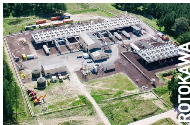
Figure 4: Rotokawa geothermal plant, a combined cycle flash-steam/binary station (photo: Mighty River Power).
