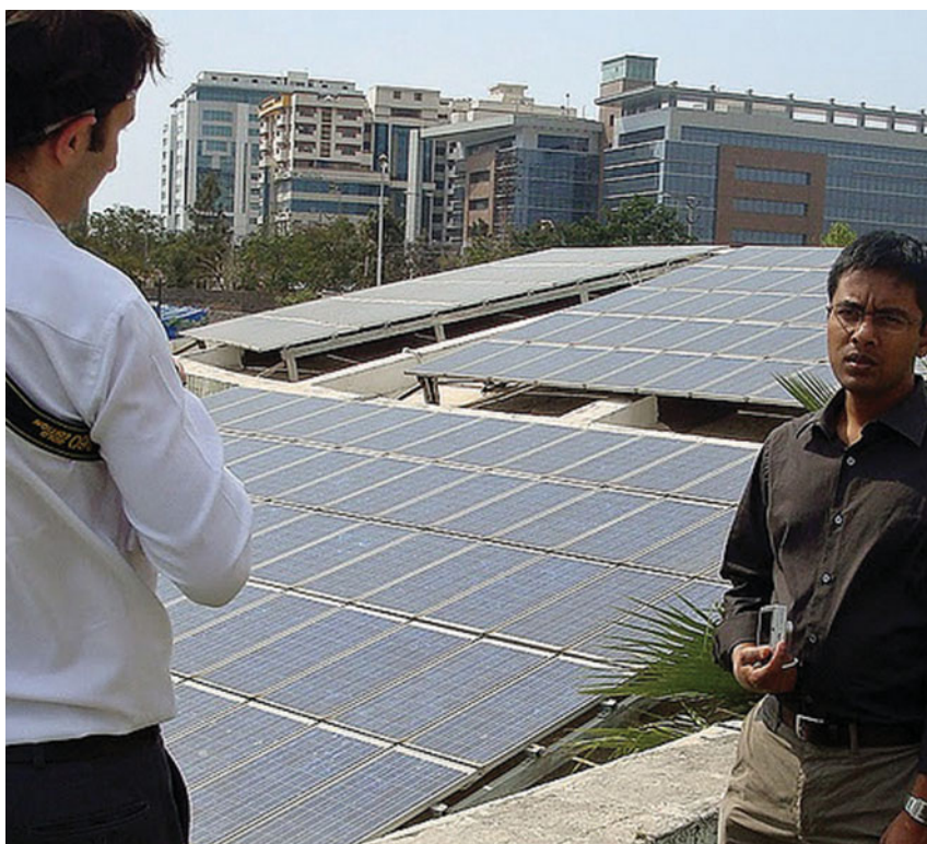
Solar panels on the roof of the Confederation of Indian Industry's Godrej Green Business Center in Hyderabad. Credit: Natural Resources Defense Council
