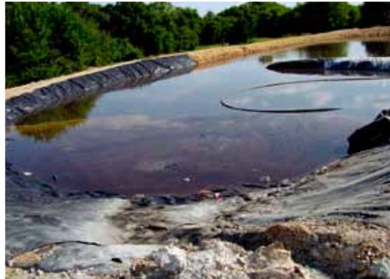
Braden Exploration waste pit just feet from a creek that flows into Denton Creek, Wise County. Photograph by Sharon Wilson.
