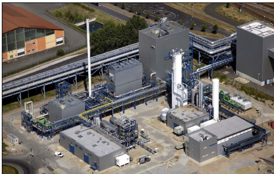
Figure 22. Oxy-Combustion Pilot Plant Capturing CO 2 from the Flue Gas of a Coal-Fired Boiler at the Schwarze Pumpe Power Station in Germany
