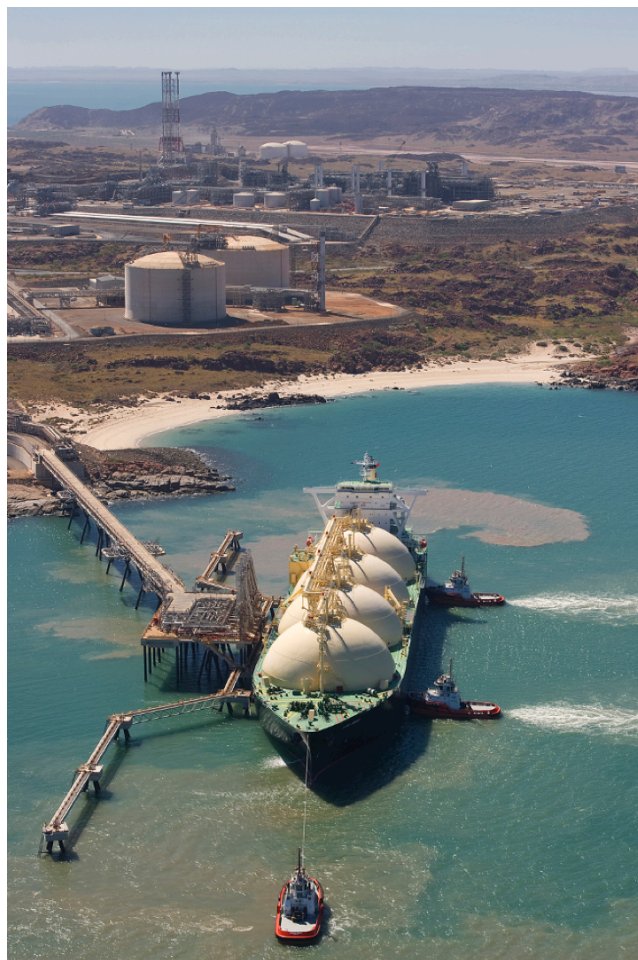
LNG facility in Australia
