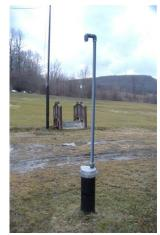
A variety of vented caps are available from most well drillers for less than \$100. Be sure to install these caps correctly to prevent insects and small animals from entering the well. Most have a screen and are turned down. You also want to have the vent tall enough to avoid any potential combustion situations, such as a passing lawn mower (picture courtesy of Susan Gohr, Twin Lakes Water Treatment, Lawrenceville, PA).
