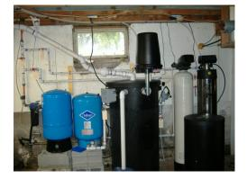
A typical aeration treatment unit installed to remove dissolved methane from a water well supply (picture courtesy of Susan Gohr, Twin Lakes Water Treatment, Lawrenceville, PA)
