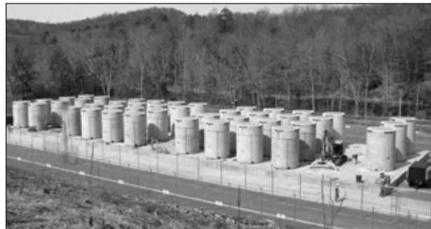
FIGURE 6 Independent spent fuel storage installation (ISFSI). Used with permission of NAC International, Inc.
