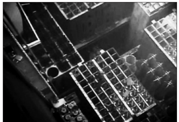
FIGURE 3 The robust construction of steel-lined concrete storage pools protected used uranium fuel rods even though hydrogen explosions ripped through the secondary containment buildings at three reactors at Fukushima Daiichi. Source: Tokyo Electric Power Company. Available online at http://www.tepco.co.jp/en/news/library/movie-01e.html .
