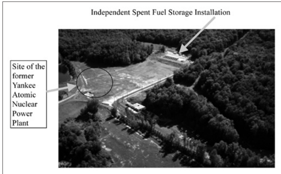
FIGURE 9 Decommissioned Yankee Atomic Electric Company site with ISFSI. Source: Yankee Atomic Electric Company.
