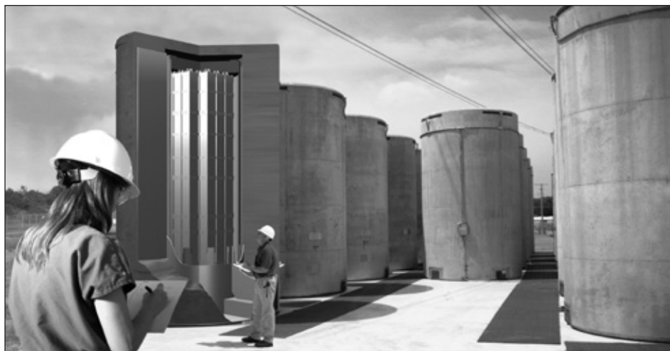
FIGURE 4 As used fuel storage pools reach capacity, energy companies are moving used uranium fuel rods to dry container storage for long-term storage at reactor sites.
