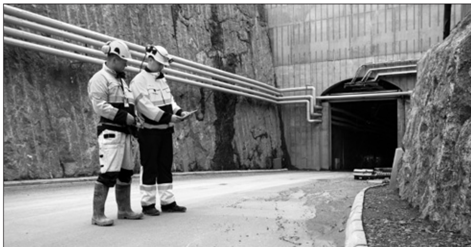
FIGURE 5 The Onkalo repository is a huge system of underground tunnels in Finland that is being hewn out of solid rock. The facility is being designed to protect the environment for 100,000 years. Source: Posiva Oy. Available online at http://www.posiva.fi/en/databank/image_gallery?gfid_1042=94&gpid_1042=1851#gallery_1042 .
