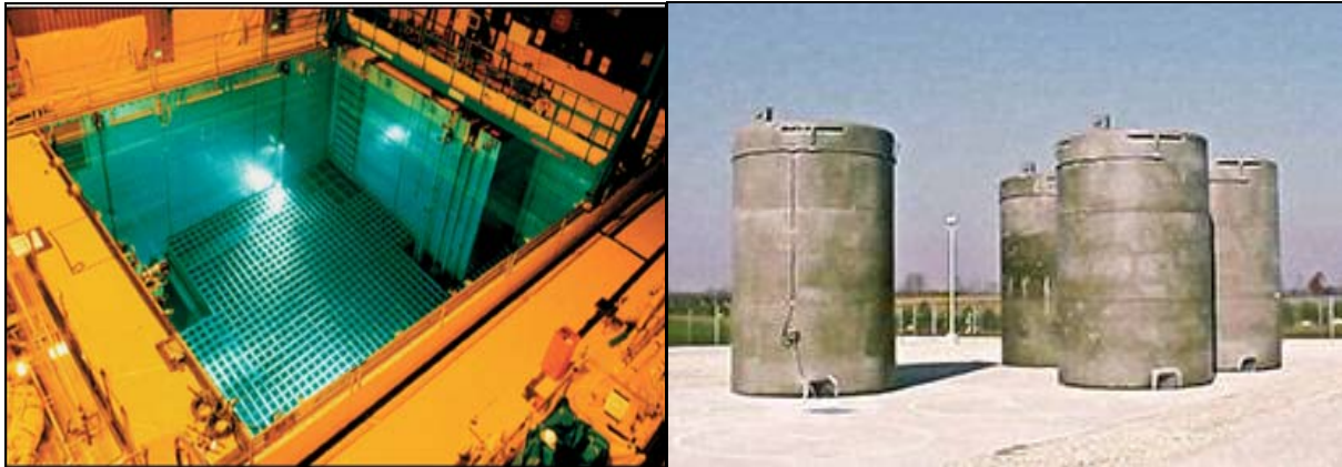
Spent Fuel Pool
