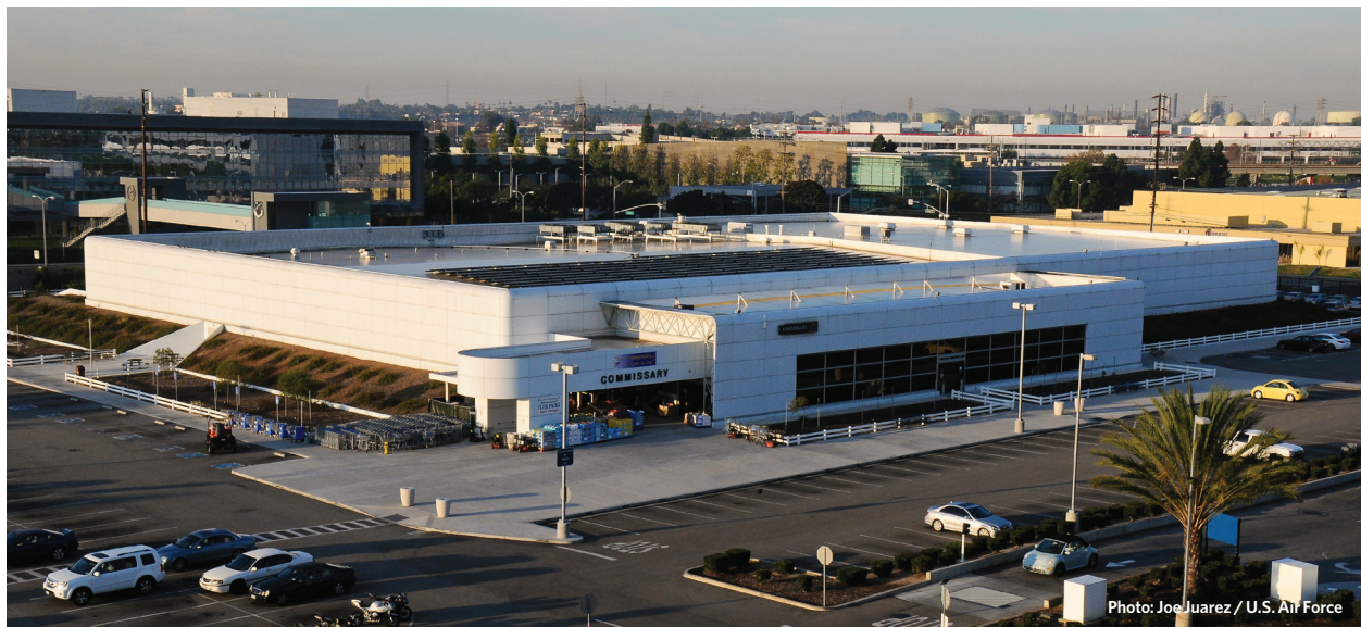
Solar panels line the roof of the commissary building at Los Angeles Air Force Base, CA, in 2011. Installation of the panels was part of ongoing energy conservation efforts on base.
