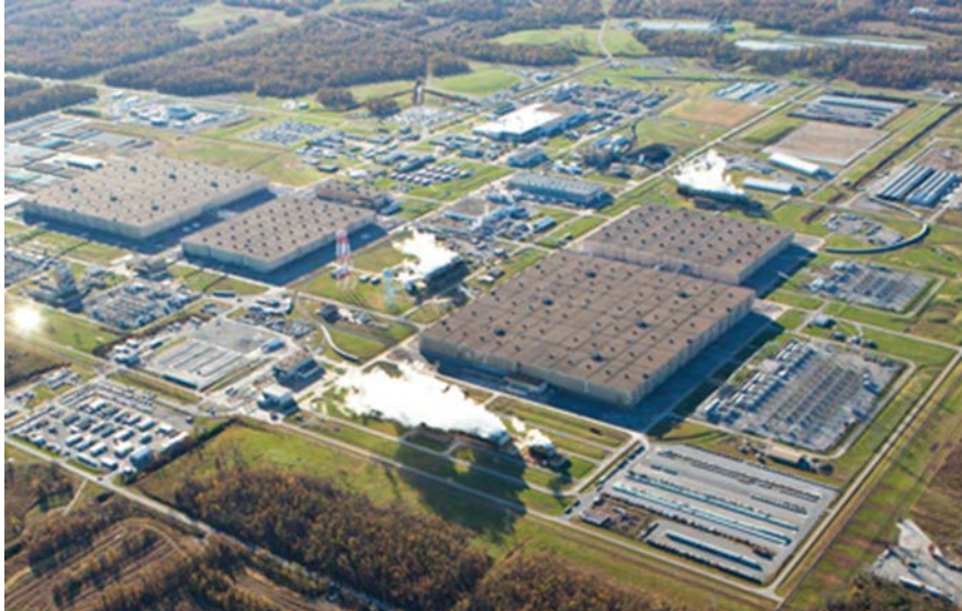
Paducah Gaseous Diffusion Plant
