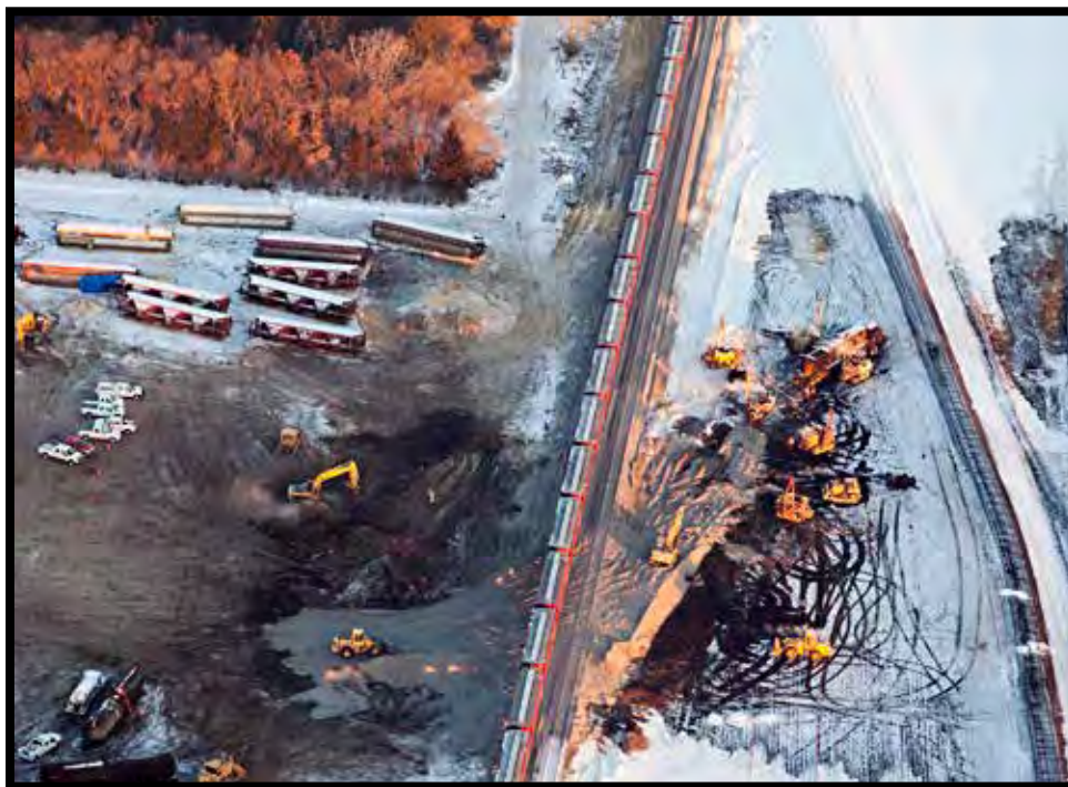
Figure 4 Casselton, North Dakota Oil Train Derailment
