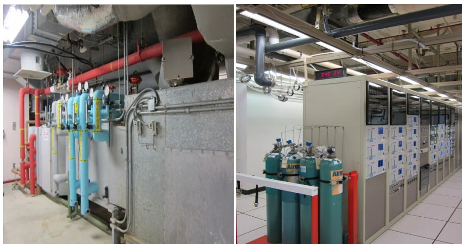
The turquoise, gray and red pipes are used to control the airstream conditions, temperature and humidity in a test chamber (left) and a bank of analyzers used for pollutant monitoring (right). (EPA OIG photos)
