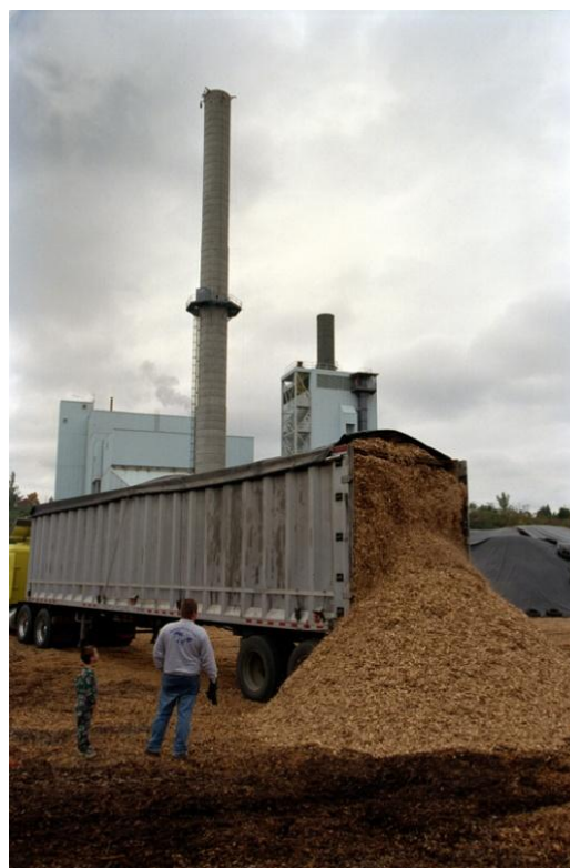
Figure 8. A 50 MW bioenergy plant burns the equivalent of a truckload of chips approximately every 20 minutes. Photo credit: NREL.
