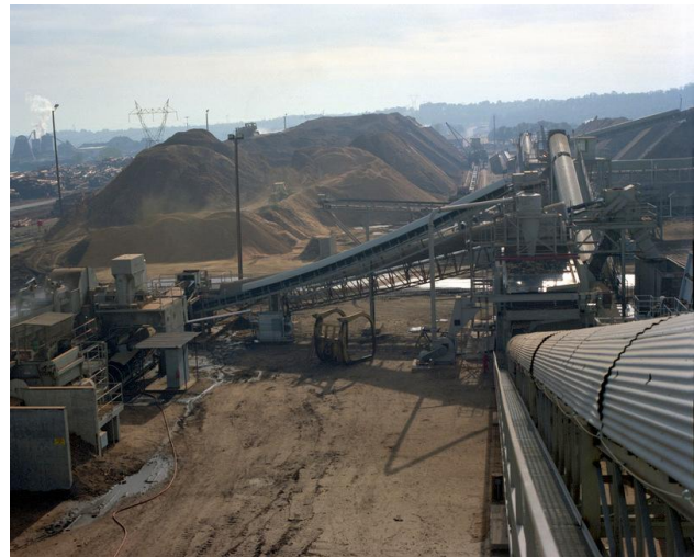
Figure 3. The massive woodchip fuel pile at a 49-MW bioenergy plant in California. (Photo credit: NREL)
