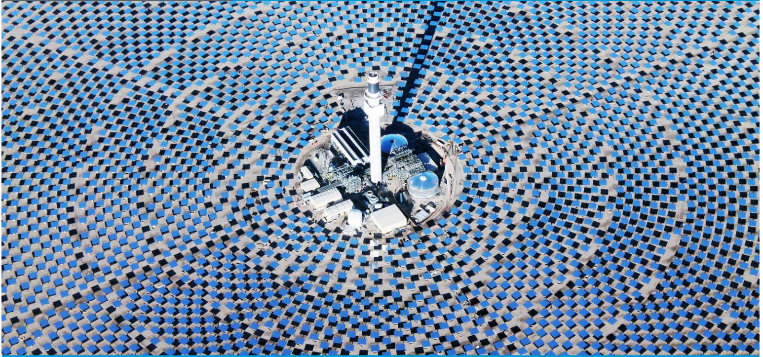
Aerial view of the Crescent Dunes 540 foot power tower in Tonopah, Nevada. Photo Credit: SolarReserve, LLC.
