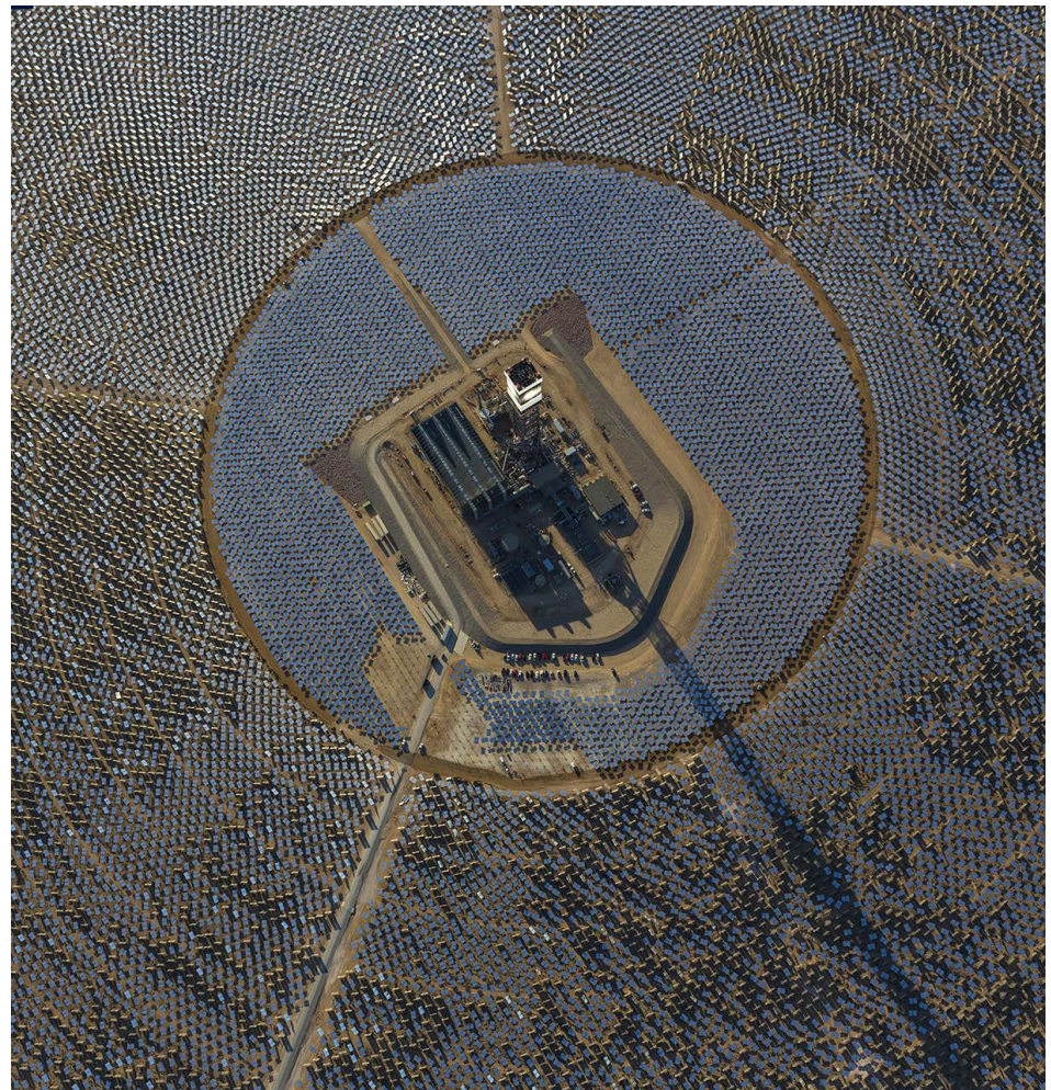
Aerial view of one of the Ivanpah power towers in Ivanpah Dry Lake, California. Photo Credit: BrightSource Energy
