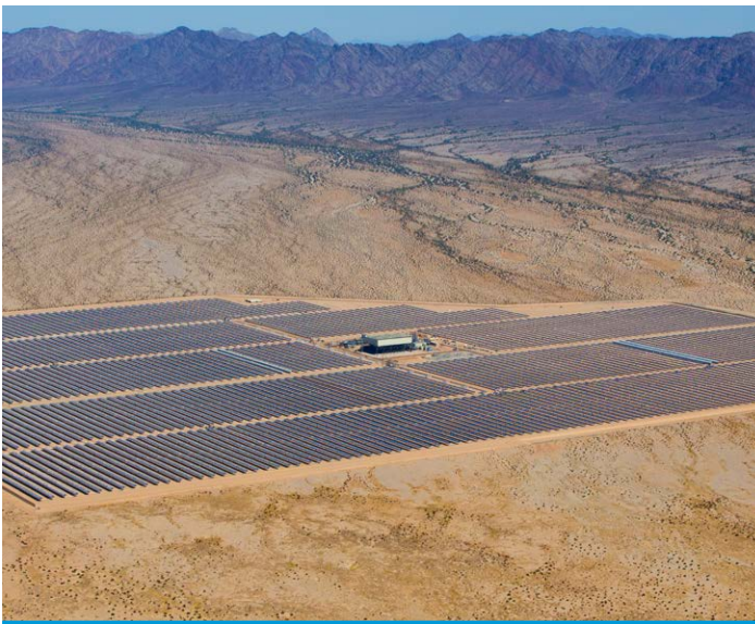
The Genesis solar energy plant is composed of two 125 megawatt parabolic trough technology units.
