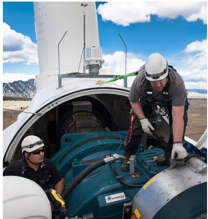
Siemens employees work on the nacelle of a 2.3 MW wind turbine in Boulder County, Colo.
