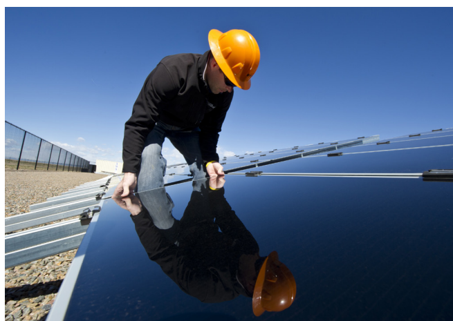
A SunEdison engineer lays a solar panel in Colorado.
