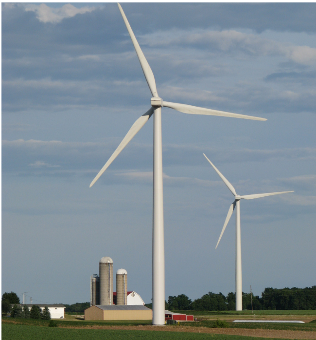
Wind turbines at the Forward Wind Energy Center in Fond du Lac and Dodge Counties, Wisc.
