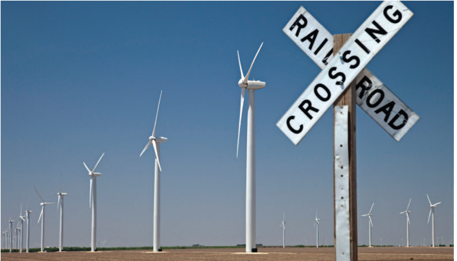
image RAILROAD CROSSING SIGN AT ROSCOE WIND FARM, TEXAS. THE 627 WIND MILLS ARE PRODUCING 781 MEGAWATT, WHICH IS ENOUGH ENERGY TO SUPPLY A QUARTER MILLION HOUSEHOLDS IN TEXAS.
