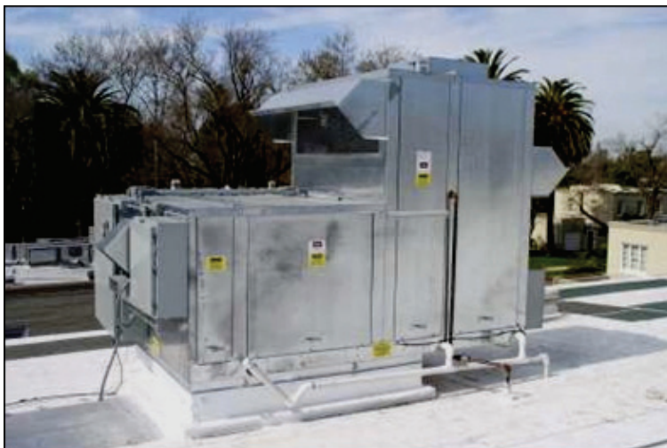
Prototype Installation of DEG's HyPak Rooftop HVAC System
