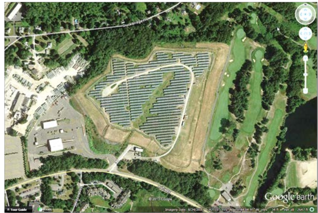
Scituate Landfill solar installation (August 2013). Courtesy of Google Earth
