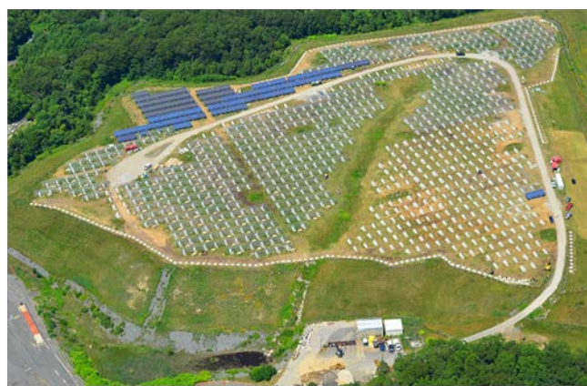
Scituate Landfill solar under construction. Courtesy Brightfields Development LLC
