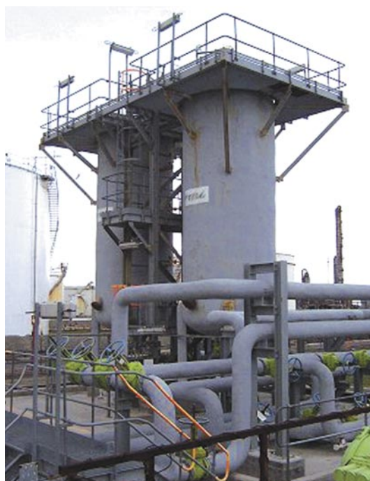
Example of a mercury removal unit (MRU)
