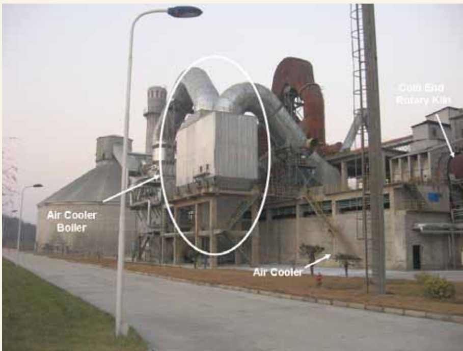
Figure 6: Air Cooler Waste Heat Boiler
