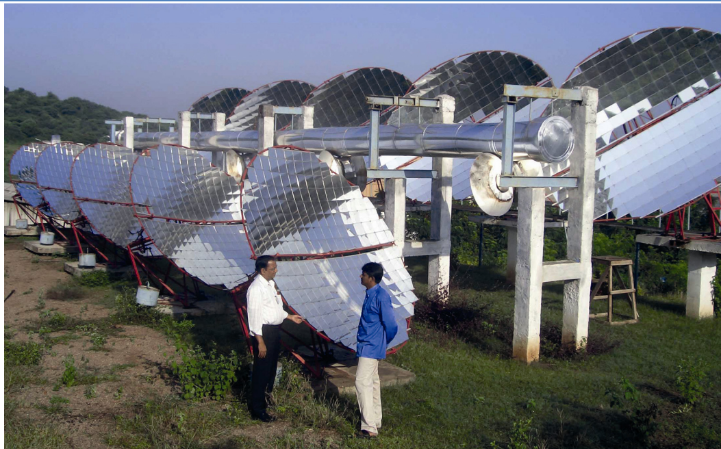
Figure 21 • Scheffler dishes associated in pairs in a cooking system at Hyderabad (India)
