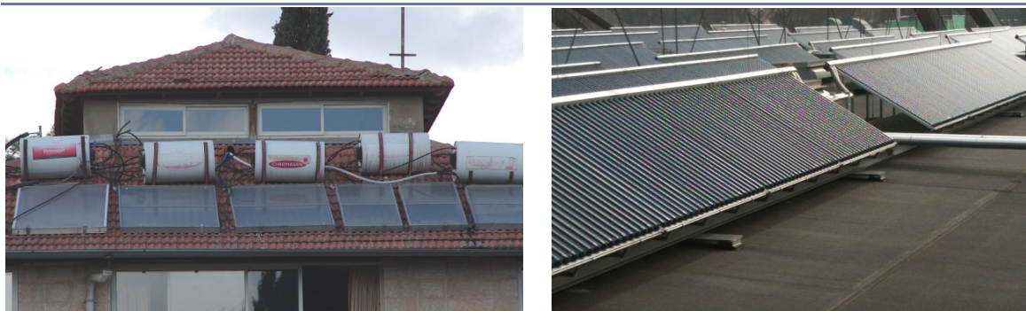
Figure 19 • Solar hot water system with flat-plate collectors on a rooftop in Jerusalem, Israel (left), and 2 MW th solar thermal system using evacuated tubes to provide district heat in Wels, Austria (right)
