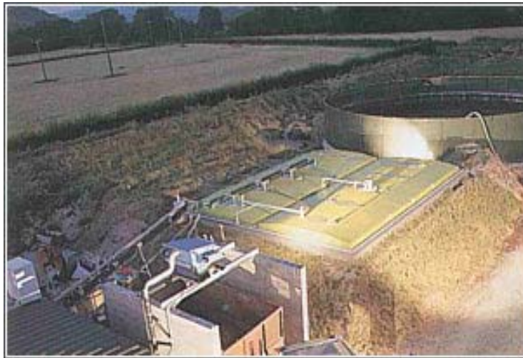
Figure 7-5 Waste Works Facility 177
