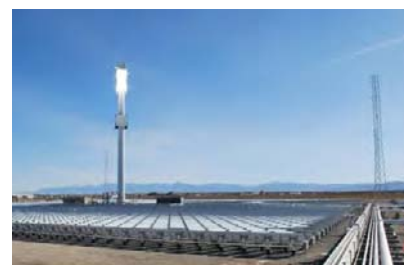
Diffuse glare from the central receiver of a solar power tower Image courtesy of Recharge News.
