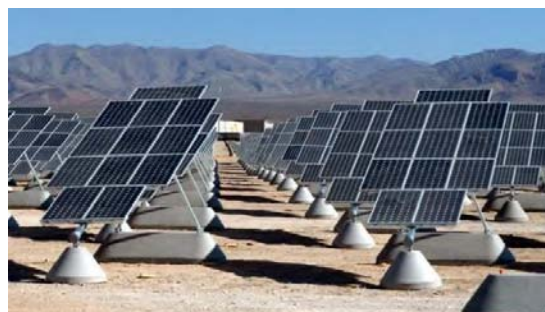
Nellis AFB Solar PV on Single-Axis Trackers Image courtesy of Gizmag.
