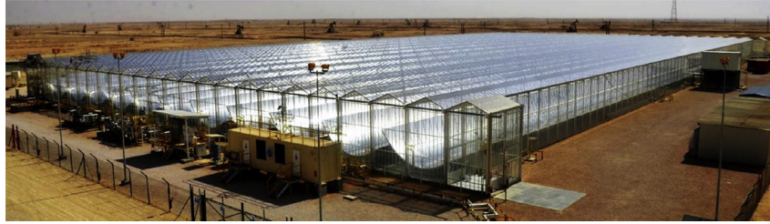
Fig. 2. A 7 MW GlassPoint solar thermal installation in Oman [26].
