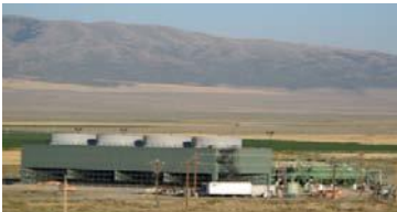
Raft River Geothermal Plant in Idaho
