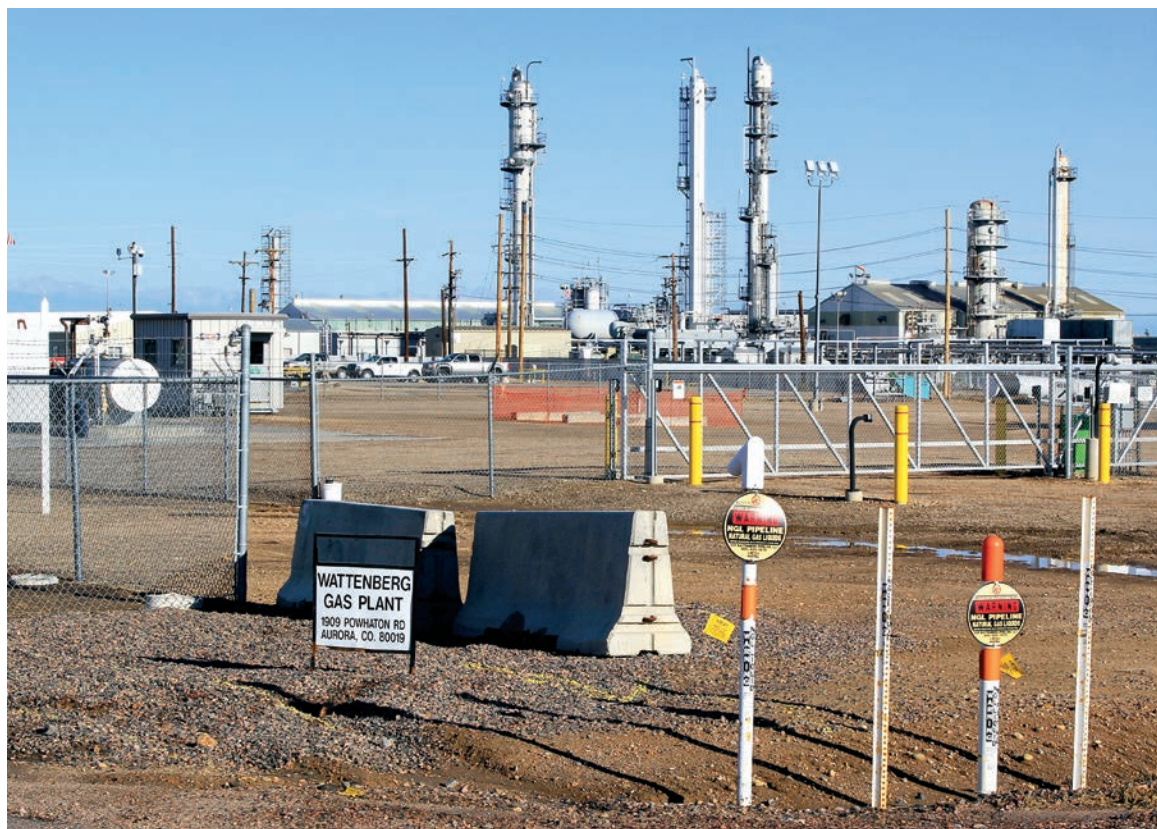
Natural gas processing plant in the Denver-Julesburg Basin in Colorado. Gas processing is responsible for 11 percent of methane emissions.
