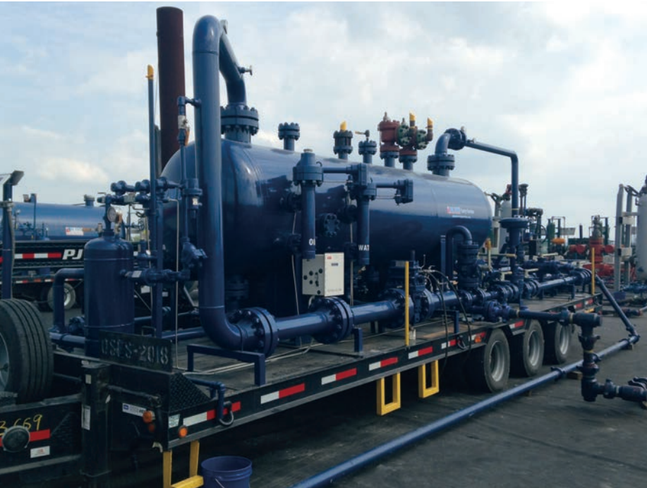
Reduced emission completion equipment at hydraulically fractured natural gas well in Washington County, Pennsylvania. EPA's 2012 standards required operators to use Reduced emission completion equipment during natural gas well completions, which significantly reduces emissions during this process. However, completions at hydraulically fractured oil wells were not covered by this requirement.
