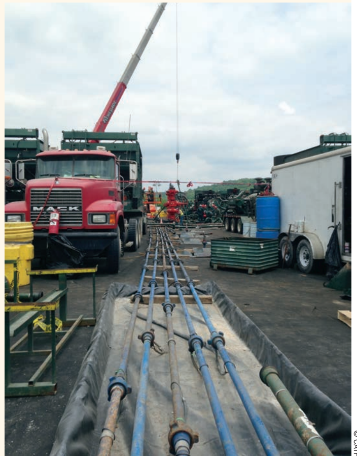
Hydraulic fracturing equipment at a natural gas well in Washington County, Pennsylvania.
