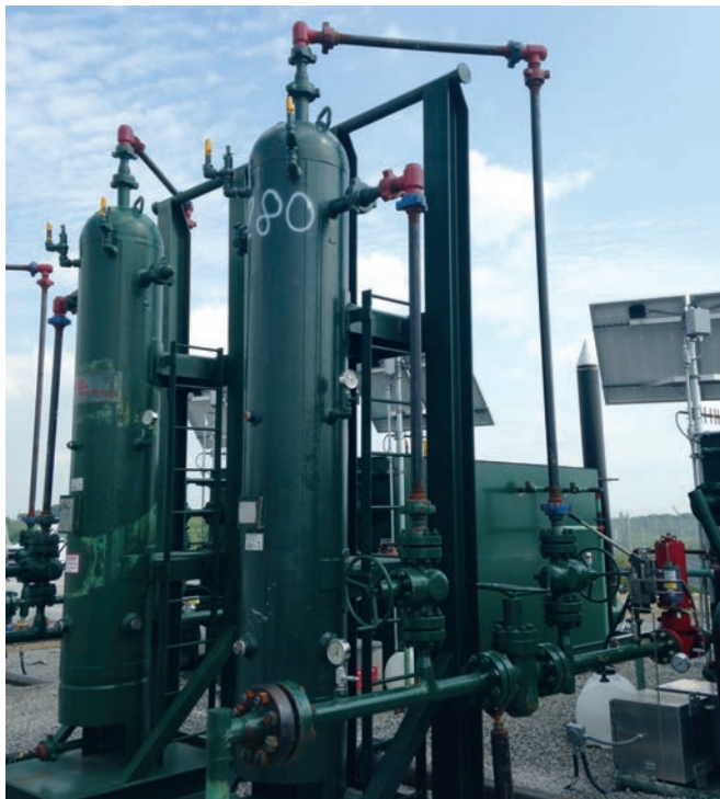
Sand traps at a natural gas well in Washington County, Pennsylvania.
