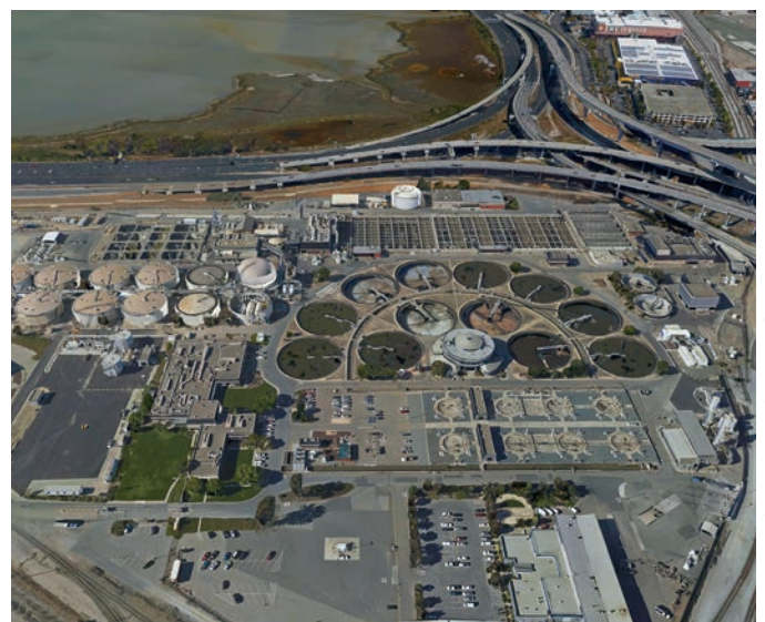
The East Bay Municipal Utility District's wastewater treatment plant in Oakland is a net producer of electricity.
