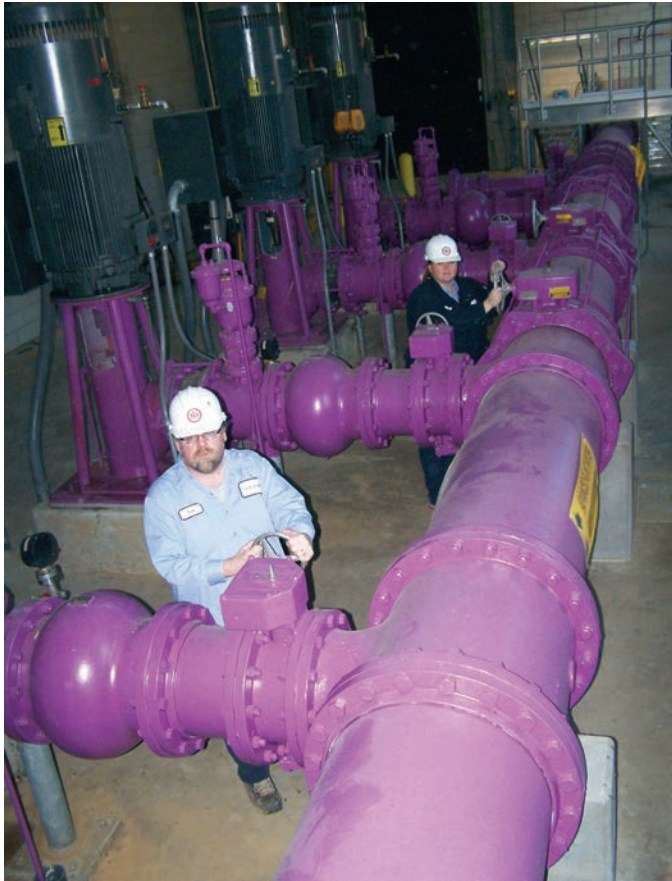
The water sector's electricity needs are growing due to drought, increasingly stringent federal water quality standards, and more energy-intensive water supplies such as recycled water. Recycled water is delivered through the purple pipes seen here.
