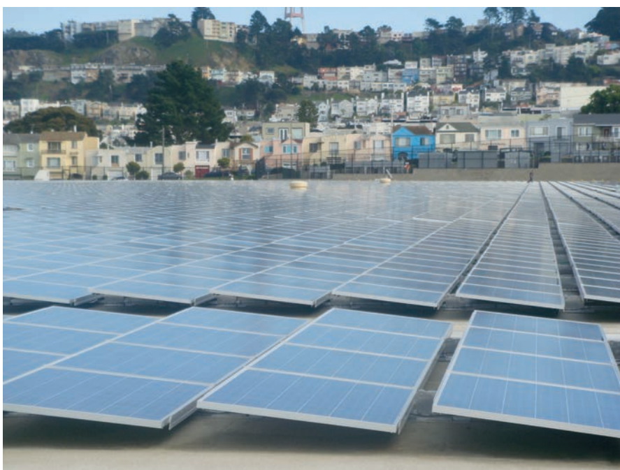
In 2010, the San Francisco Public Utilities Commission completed construction of a 5 MW solar photovoltaic installation on the roof of Sunset Reservoir.
