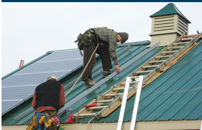
Workers install 6,800 watts of PV solar panels on the Kilpatrick Farm in Warren, OH. (Photo courtesy of Dovetail Solar and Wind)
