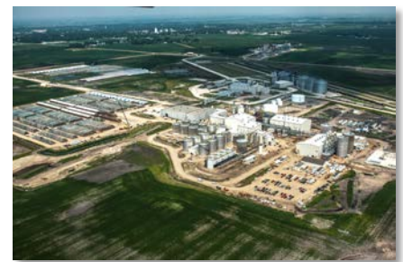
POET's Project Liberty cellulosic ethanol facility in Emmetsburg, IA, which began production in September 2014. Photo courtesy of POET.
