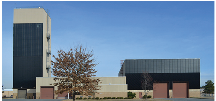
The solar wall at Fort Bragg's "rigger shed" uses a solar wall that helps circulate warm air through the tall structure, helping to dry parachutes used by the 82nd Airborne.
