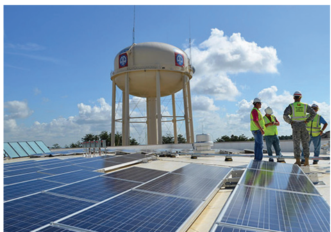
A rooftop solar PV array at Fort Bragg in North Carolina.
