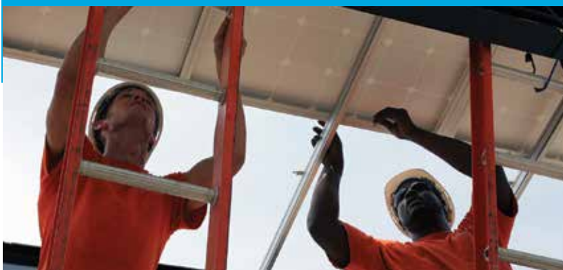
Brightergy employees install a solar canopy in Kansas City’s West Bottoms district. (Photo courtesy of Brightergy)
