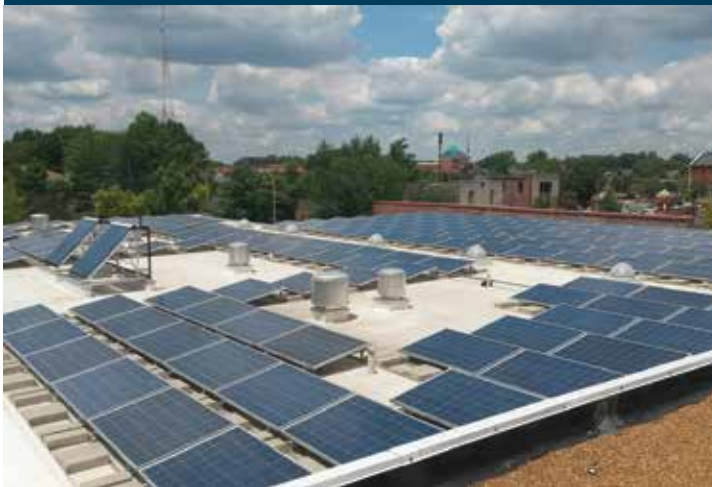
The solar array at Crossroads College Prep School in St. Louis was installed by StraightUp Solar. (Photo courtesy of StraightUp Solar)
