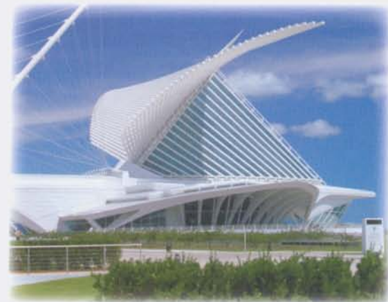
The Milwaukee Art Museum incorporated high volume fly ash concrete to achieve a variety of important design objectives.
