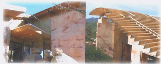
This residence designed by Arizona architect, Michael Frerking utilizes 67 percent fly ash concrete.
