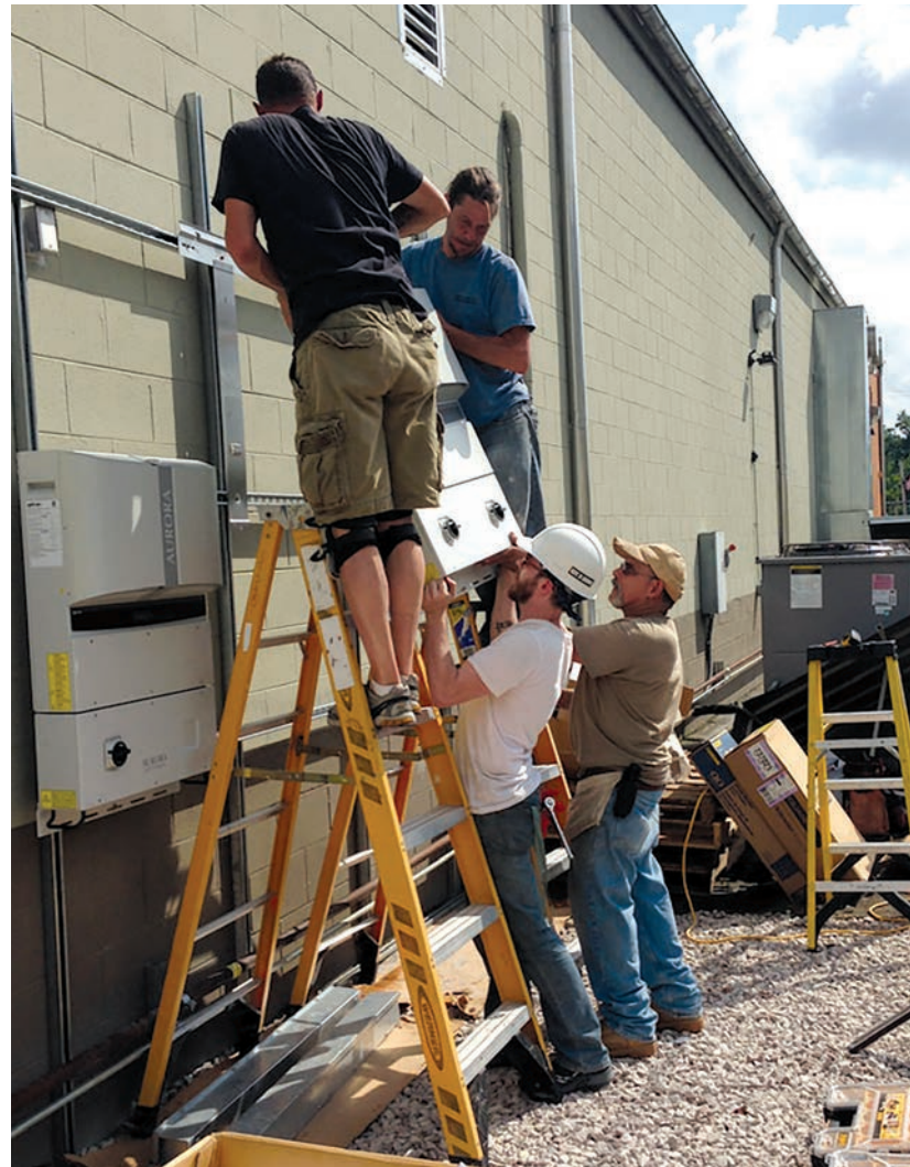
Workers install equipment at the Three Rivers Market in Knoxville. (Photo courtesy of ARiES)
