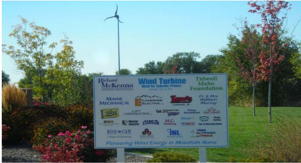
Figure 10. Turbine at Richard McKenna Charter High School in Mountain Home, Idaho. Photo from Todd Haynes, NREL/PIX 18602
